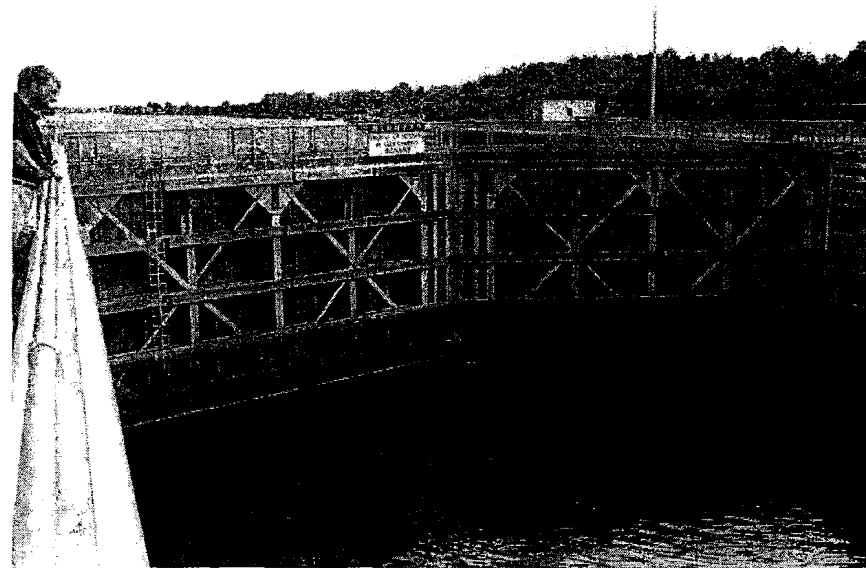
Photo 4-10: Inglis Lock – Head Gate
